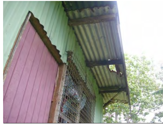
replacing roofing iron above bedroom area
