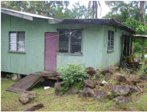
Construction of new ramp and safety guide
